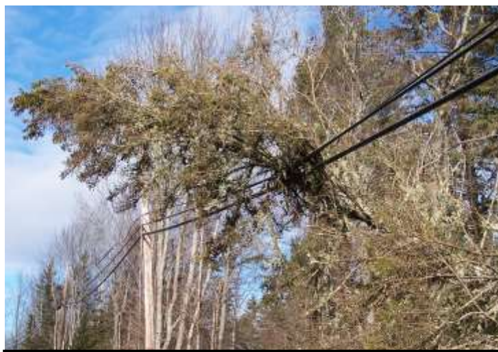
This tree on Buttermilk Road broke the power lines feeding the eastern end of the road. Emera Maine eventually removed the hazards.
