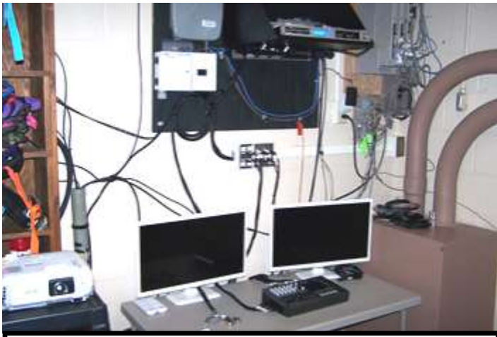
The TV switching equipment at the Lamoine School
