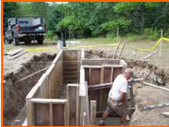
Concrete contractor Allen Doll sets the forms
