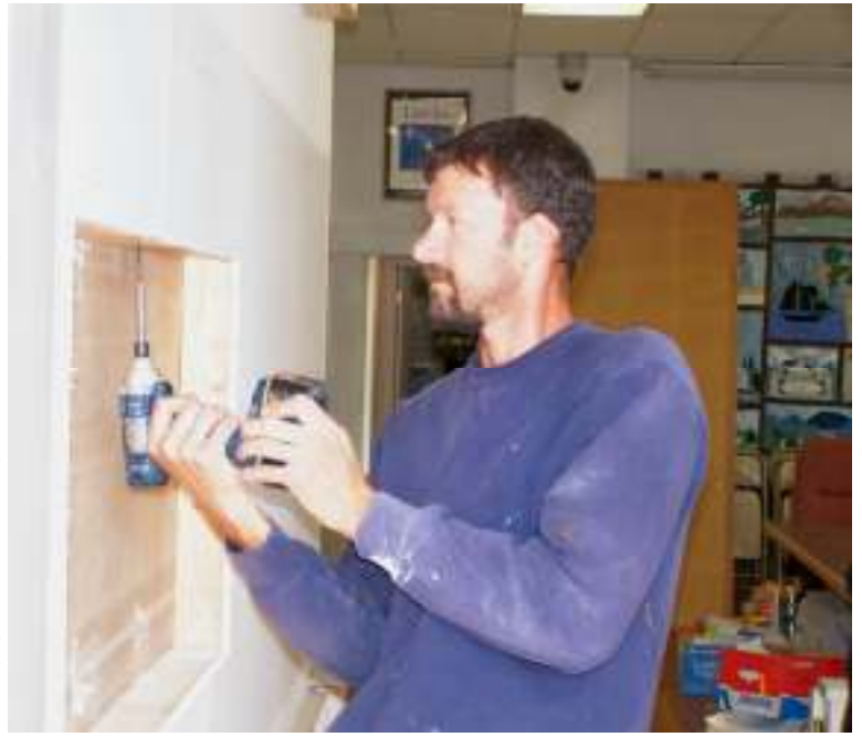
Matt Randall of AA Randall & Sons installs the frame for the new window in the Administrative Assistant's Office
