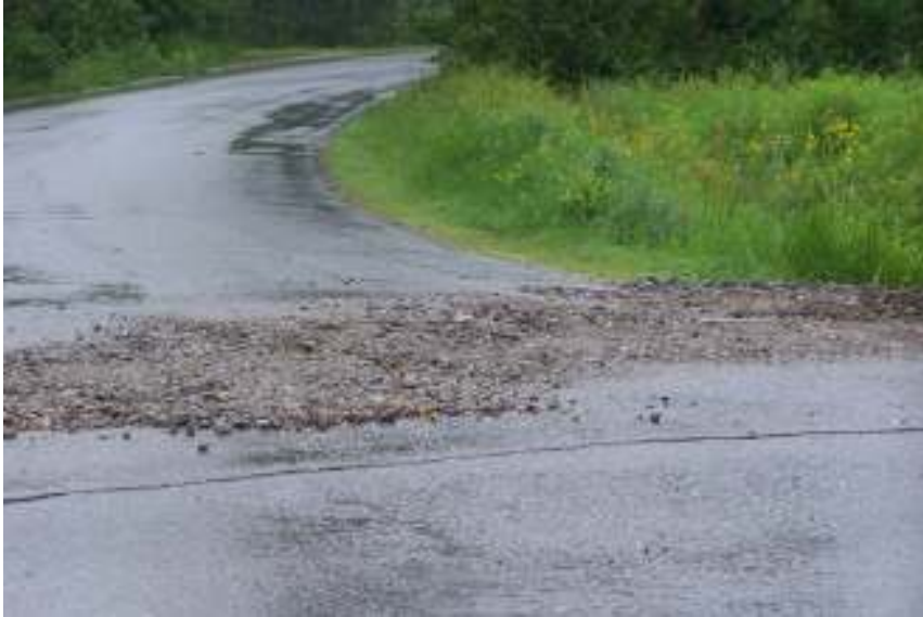
Culvert fill @ Raccoon Cove Road
