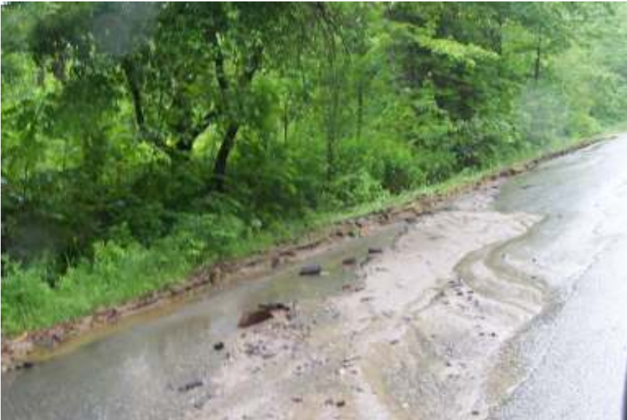
Area west of Birchlawn Drive with shoulder erosion
