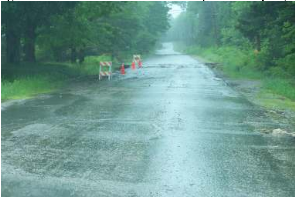
View looking toward Birchlawn Drive –barricades set up by Fire Dept.
